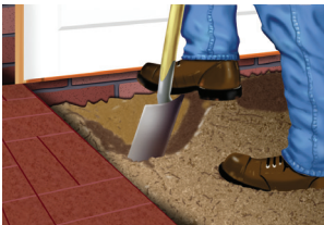
Dig trench 110mm wide by 156mm deep for channel.
