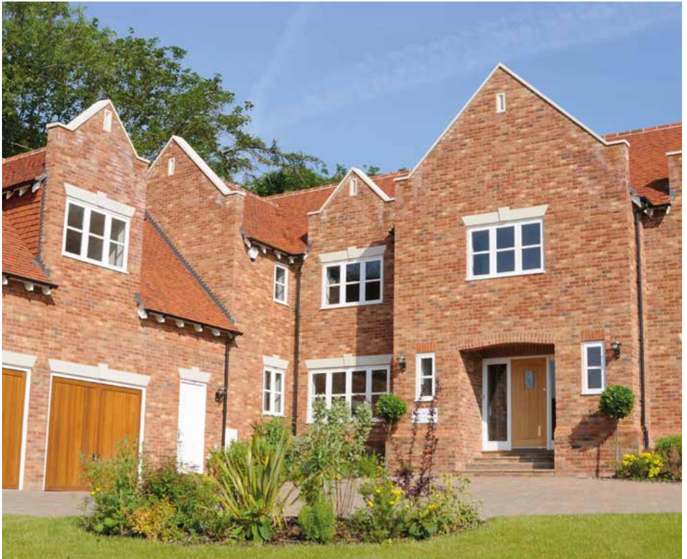
Private residence OLDE FARDALE MULTI
