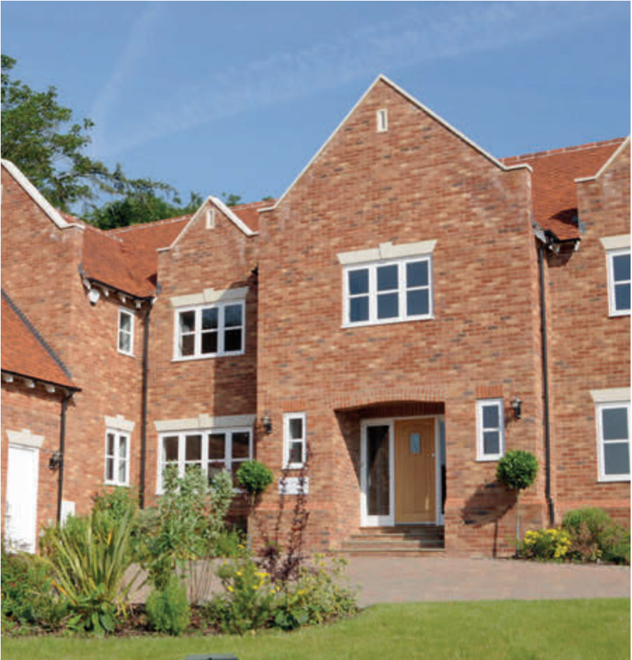
Private residence OLDE FARDALE MULTI
