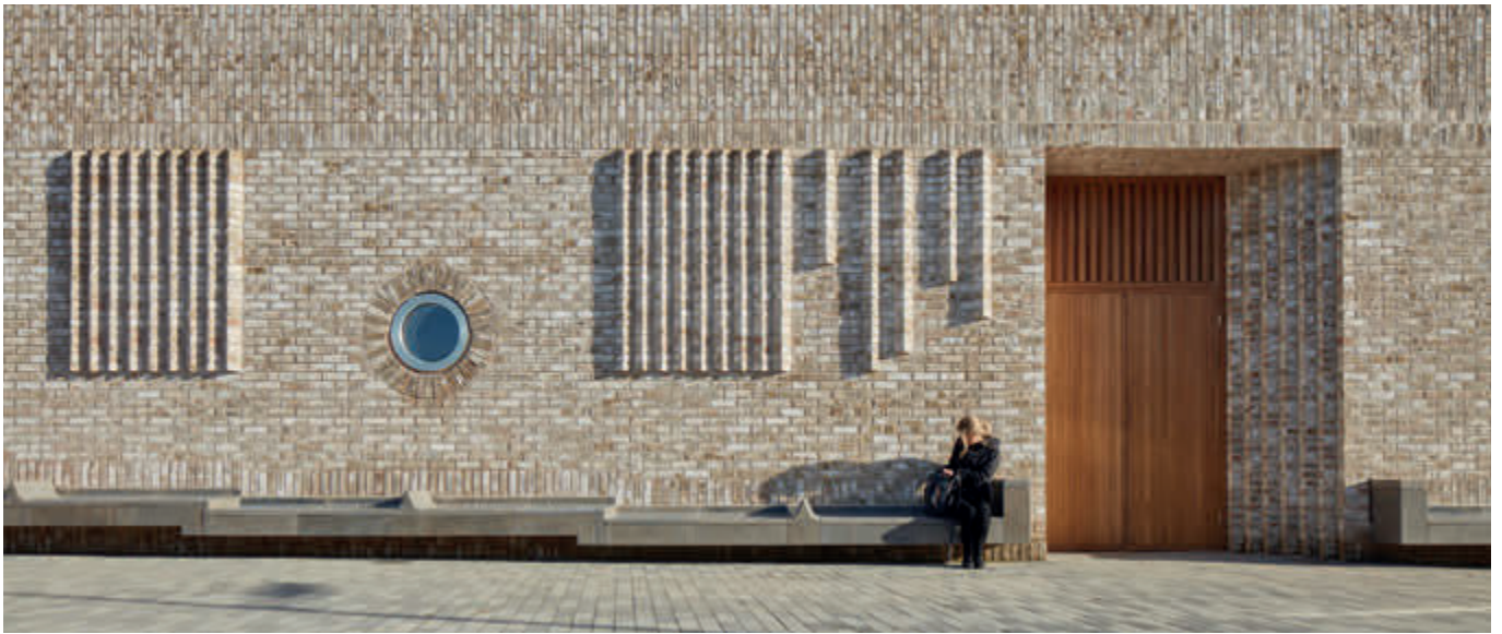
Storey's Field Community Centre and Nursery, Eddington, Cambridge CON MOSSO
