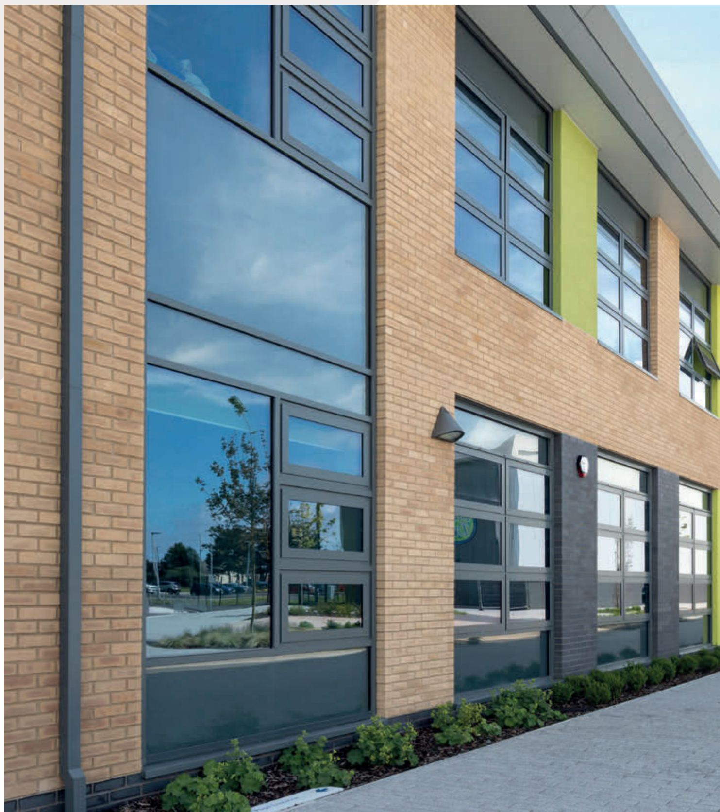
Ysgol Gymraeg Bro Dur, Sandfields, Port Talbot BROOKHURST YELLOW AND STAFFORDSHIRE SMOOTH BLUE
