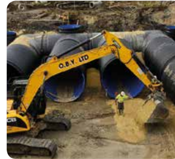
Yorkshire Water utilises largest diameter Ridgistorm-XL for Section 104 trial scheme
