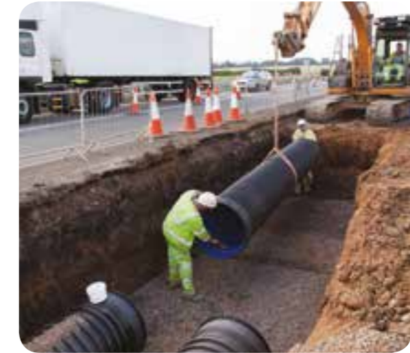
Vital road improvement project relies on Ridgistorm-XL
