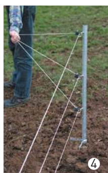
4 Run the polywires over the corner insulators at the corners
