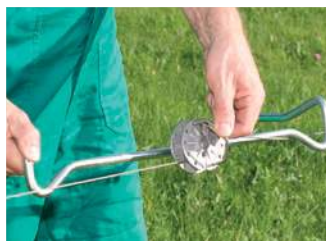
Hang the wire tensioner handle in the wire, install the cotter pin and remove the wire tensioner handle.
