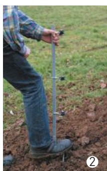
2 Set corner posts at all corners and curves
