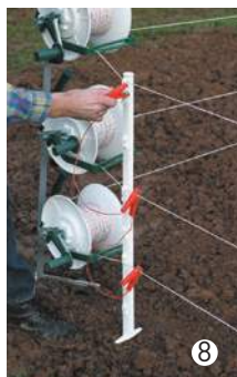
8 Attach the cross-connection approx. every 200 m
