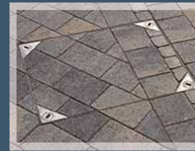
Blocks mortared into position around a cover
