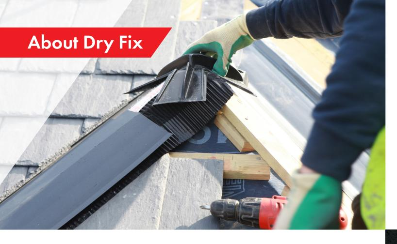
Dry Fix is a method of mechanically fixing Ridge and Hip and Verge. As well as additional components such as valley troughs and bonding strips, which traditionally have been fixed with mortar. The majority of roofs in the UK are now completed using Dry Fix components, including new builds, re-roofing and refurbishment projects.
