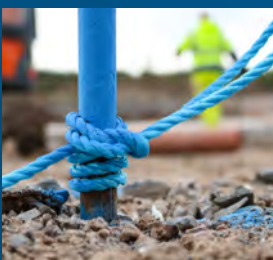
Ropes & Brick Line
