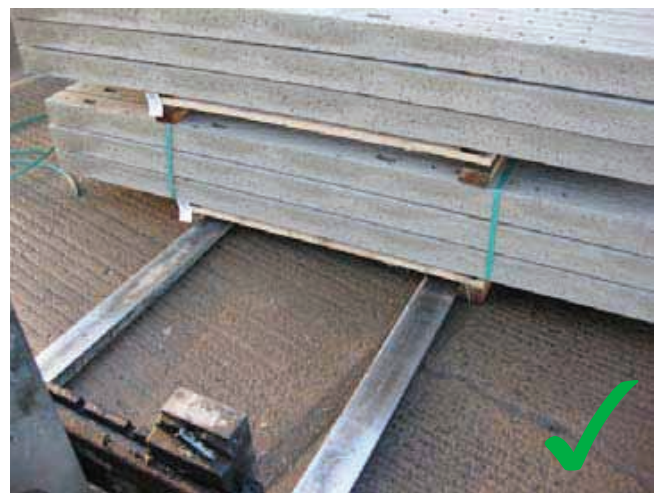
The forks MUST NOT be close together when picking up packs. The forks MUST be widened to be as close to the load bearer as possible
