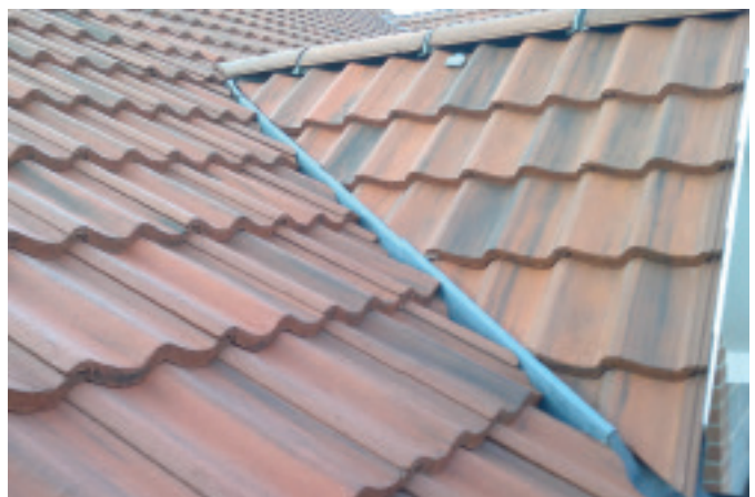
F. The completed installation: neat, tidy and effective with minimal on-site time.
