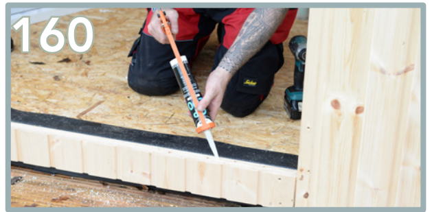
Apply the adhesive silicone in the door section. Be sure to seal the ends of sill and frame assembly to prevent moisture from tracking along the sill and into the wood work.
