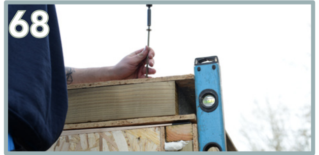
Use the spirit level to ensure the top OSB sheet of the roof panel is flush with the back edge of the wall panel. Top Tip - Use the Canopy T&G Panel (BD) as a reference for the correct overhang size at the front.
