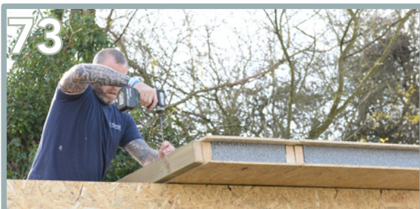
Secure the second roof panel to the front and back panels. Use 2 x 150mm screws at the back and 2 x 150mm screws at the front. Repeat steps 73-75 for the third Roof Panel (Y).
