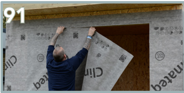
Using a Stanley knife, remove the excess from the door section, using the walls as a guide to ensure it is cut straight.
