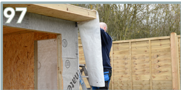
Remove the excess from each side of the roof overhang.
