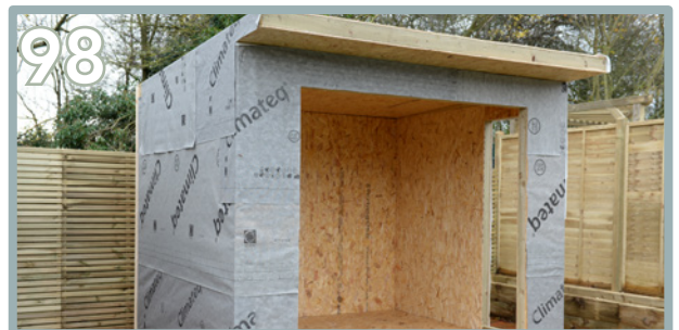
The final result is shown above. You do not need to add membrane to the canopy / the roof overhang.
