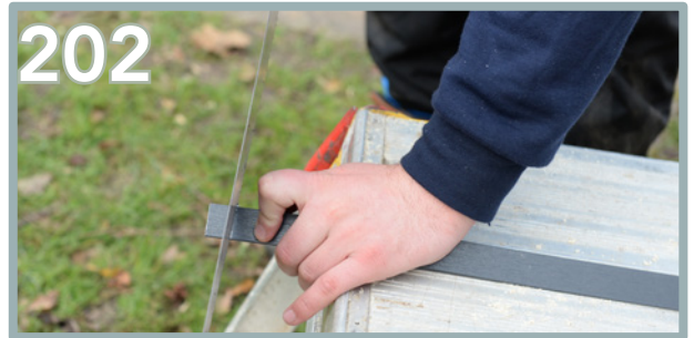
202 The side plastic trims for the door and window will need to be trimmed to fit. Mark out your required length and cut.
