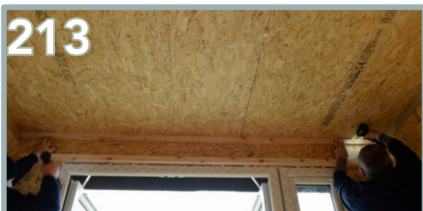
Secure one batten above the door opening, flush to the edge opening. Secure the top batten flush to the ceiling. Use 5 x 80mm screws per batten.
