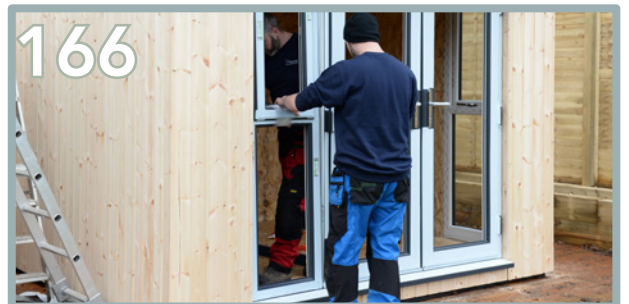
Insert the window frame into the left hand side of the double doors. The metal cap will slot into place.
