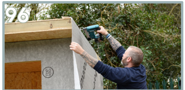
Fold onto the roof, stapling into place.
