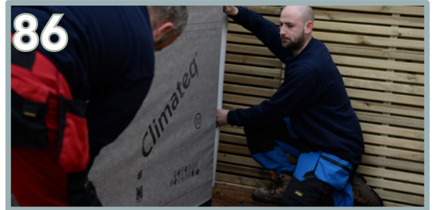
86 Continue unwrapping the membrane, pulling tightly and stapling into place.
