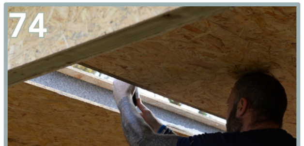
Lift up the final Roof panel (Z) and apply expanding foam into the inner groove as shown above.
