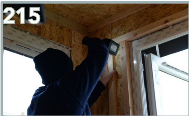
215 Using 4 x 80mm screws, secure a batten between the two added in Step 208. Repeat on the other side of the door.
