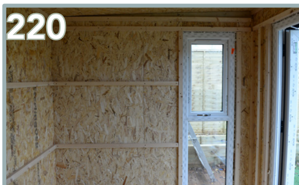
220 Use 4 x 80mm screws for each of the three smaller battens.
