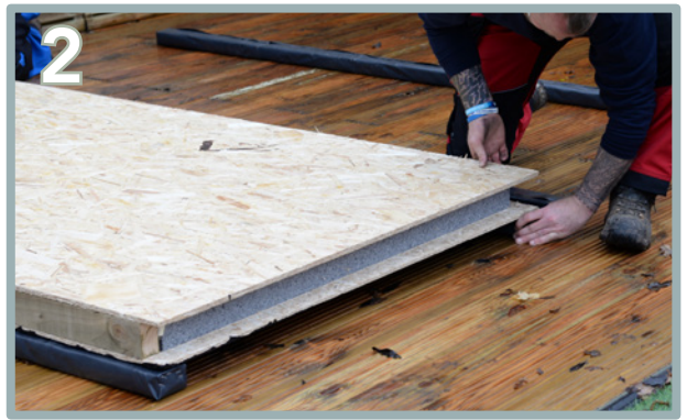
2 Place the first floor panel (D) on flush to the edge of the first bearer and halfway onto the second bearer. Place the black underside of the floor panel on top of the bearers as shown above.
