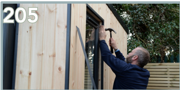
205 Pre-drill and use 5 pins down the front and 3 pins in the internal face of the side strip for the window frame. Repeat for the opposite side.
