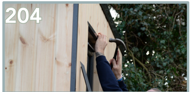
204 The same process applies for the window frame. Pre-drill and use 2 pins on the front edge and 3 pins underneath.
