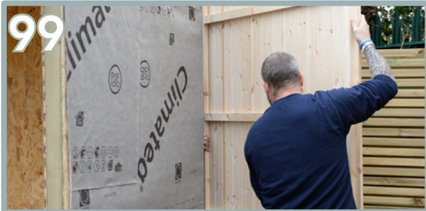
Begin applying the T&G Back Panel (AZ).
