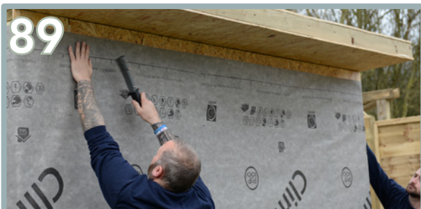
89 Add additional staples to keep the membrane in place. Be careful not to staple into the door and window gaps.
