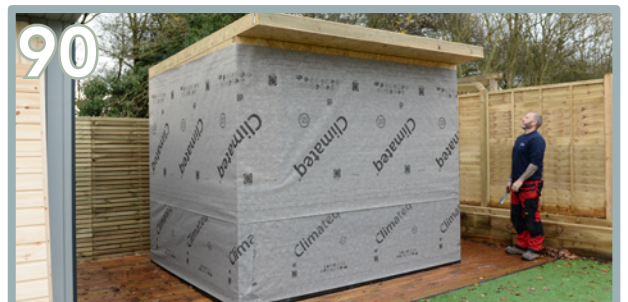
90 There will be a slight gap at the front and on the sides due to the angle of the roof.
