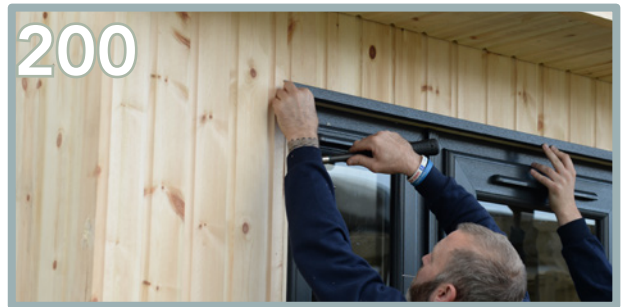
200 Using the pins provided with the trims, hammer 2 in each corner and 1 in the middle.
