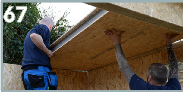
Lift up the first Roof Panel (X). Ensure at least 3 adults help carefully lift up the roof panels as they are heavy.
