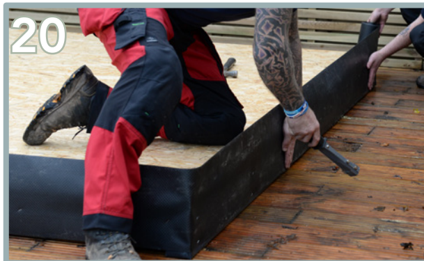
Continue to wrap around the base. We suggest one person unwraps while the other follows behind stapling the DPC into place.
