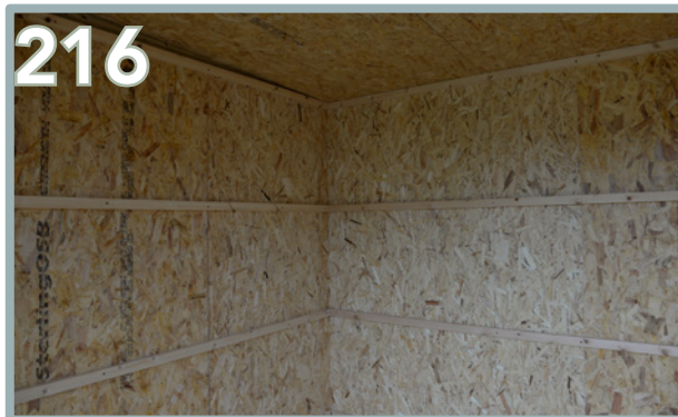
216 Secure four 45 x 28mm battens onto the left hand wall in line with and at the same height as the four back wall battens. These should be flush end to end.
