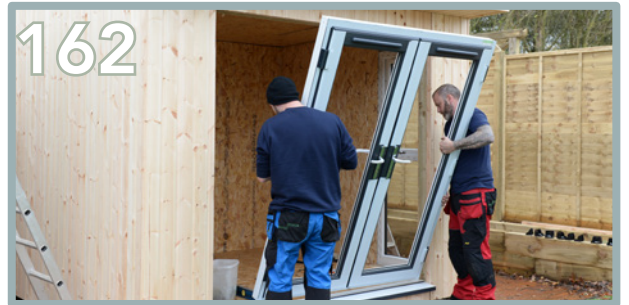
Lift and angle the frame, then insert the ledge. Butt up against the wall panel.
