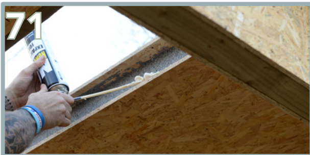
Use expanding foam in the groove of the roof panel and knock into place. Ensure the roof is flush to the front and back of the first roof panel.
