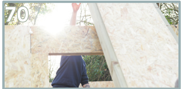
Lift and position the second Roof Panel (Y).
