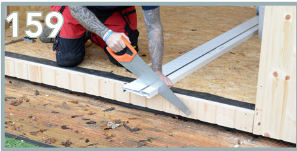
The door ledge will be oversized by 100mm. You will need to measure and cut off the excess.
