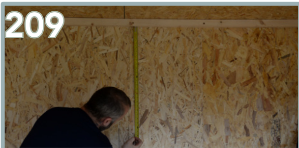
Measure and mark out even spaces to position the two middle battens.
