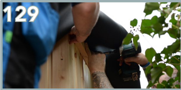
Secure the Back Roof Battens to the Back T&G Panels (AX, BI & AZ). You will need to lift up the overhanging EPDM to do this. Ensure each batten's edge is flush to the top of the T&G panel. Secure with 3 x 80mm screws per batten.
