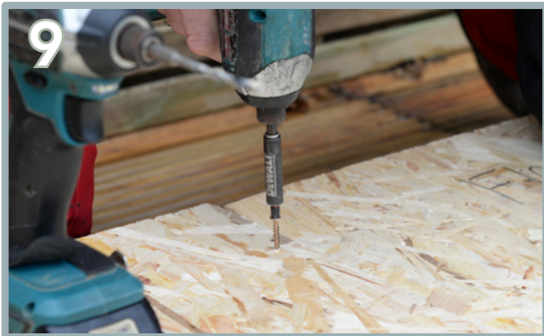
Using 4 x 35mm screws, pre-drill and screw where the adjoining panels intersect. This will secure the floor panels together. Repeat the same process for the third panel (E).
