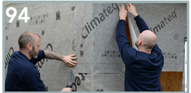
Staple into place and remove the excess from the door section.
