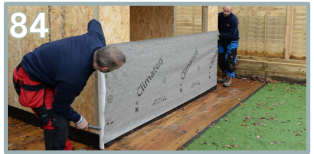
84 Starting with the bottom section, pull the membrane tightly and staple into place.
