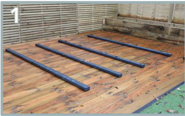
1 Lay the bearers down and spread them out roughly ready to position the floor panels on top.
