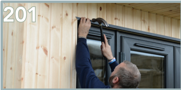
201 Pre-drill across the top and repeat the same process. Use 5 pins across the front of the plastic trim.
