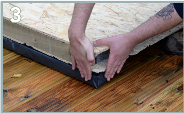
3 Ensure the panel is flush to the edges of the first bearer. Ensure the floor panel on the bearers are level using a spirit level as a guide.
