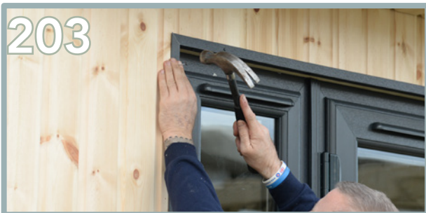
203 Use 5 pins down the front and 3 pins in the internal face of the side strip for the door frame. Repeat the same process for the opposite side.
