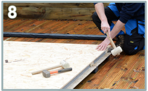
Knock on the front and back of the second panel to ensure it is flush on both edges to the first panel and floor bearers.
