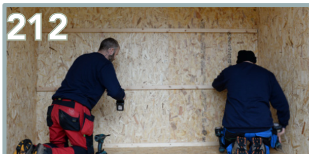
Using 5 x 80mm screws to secure into place.
