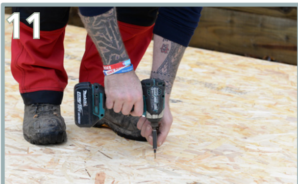
Once happy that all panels are in the correct position, further secure with 5 x 125mm screws along the outer edge of the fourth panel.
