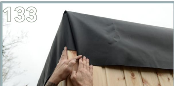
Fold the EPDM in a tucked position against the front and back of the side panels as shown above.
