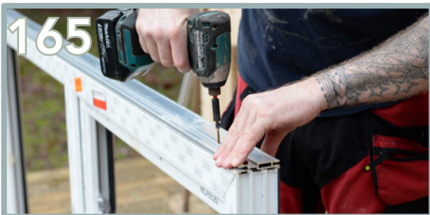
(Steps 165, 166, 169, 174, 180 and 181 are only for the 'Xtend Plus' doors and side window. These step will not apply to the standard option). Use 3 x 35mm screws to secure the metal capping.
