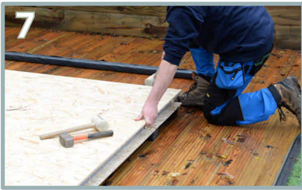
Using a rubber mallet, knock the second panel into the first for a tight fit.
