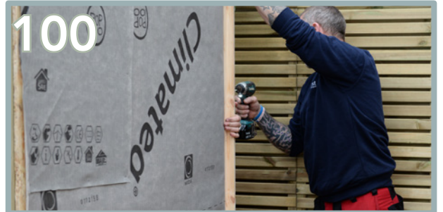
At each side, there will be a slight overhang of the T&G board. The batten's edge underneath, attached to the panel should be flush to the end. Use the 45 x 28mm batten as a guide to provide a 45mm space from the ground.
