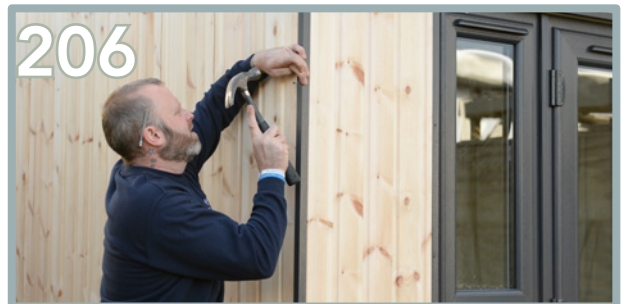
206 Add strips to each of the corners using 4 pins for each corner strip. The two back corners are shorter. Trim the strips if necessary.
