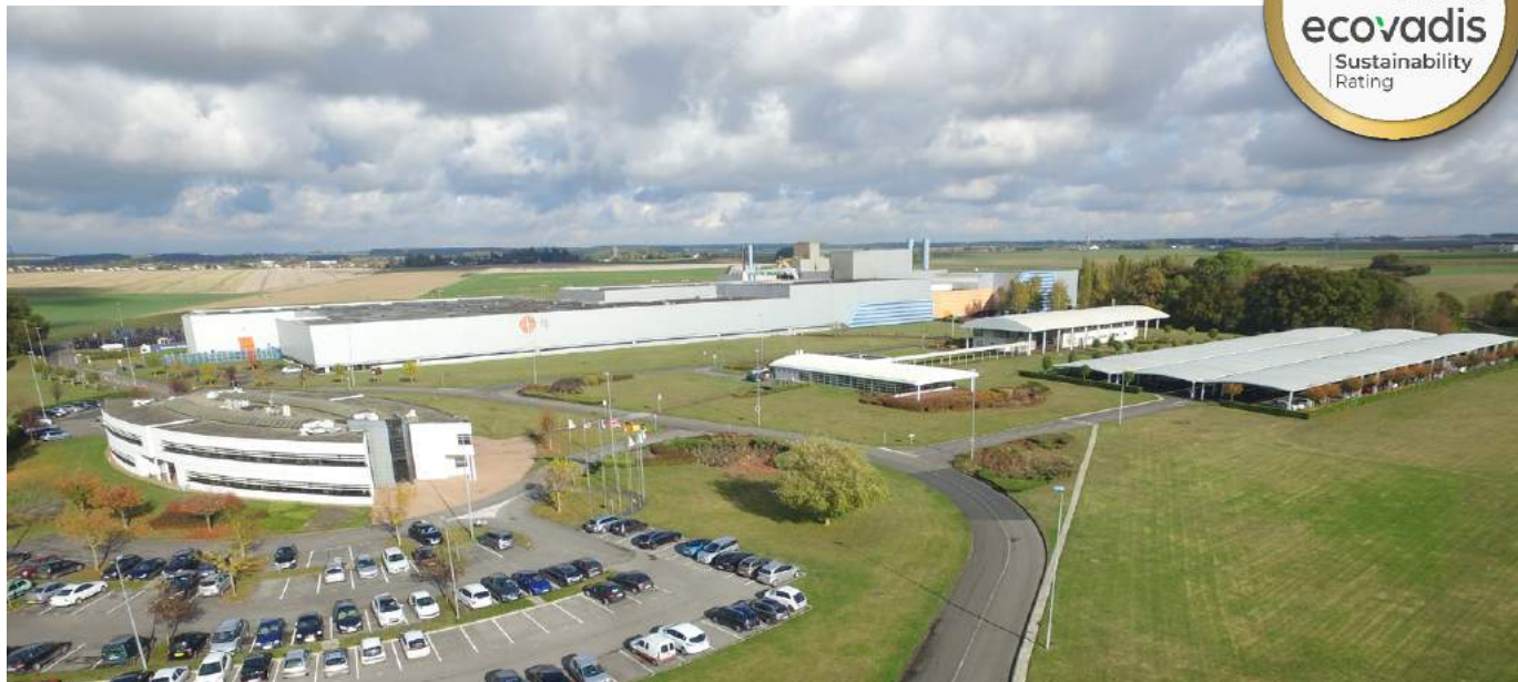
Picardie - France, the Saint Crépin Ibouvillers foundry in Oise, 723 employees, production capacity of 100,000 tonnes, 42 hectares. Management systems certified ISO 9001, ISO 14001, ISO 45001 and ISO 50001 for the management of quality, environment, hygiene, safety and energy.
