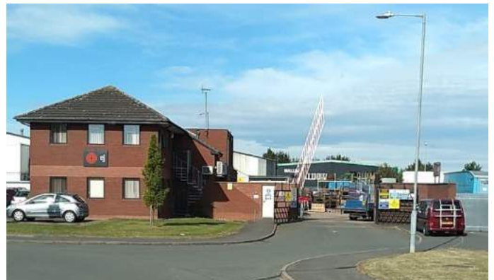
Nuneaton - UK - This is our UK distribution & manufacturing facility for galvanized and stainless steel products. Our UK facility is certified to ISO 9001 for quality management and ISO 14001 for environmental management.
