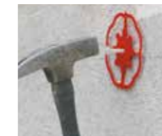
The Baunit adhesive anchors are inserted into the borehole and secured with plastic nails.
