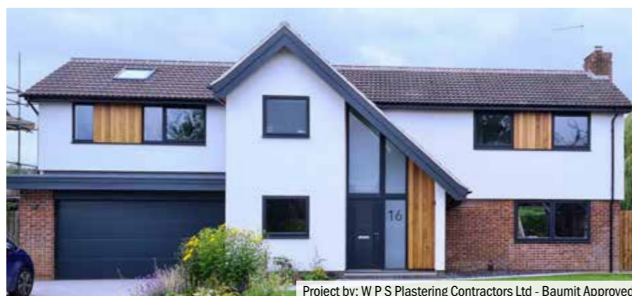
Project by: W P S Plastering Contractors Ltd - Baumit Approved
