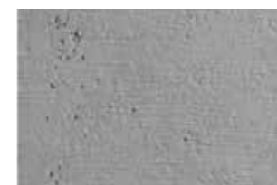
Coarse concrete technique
