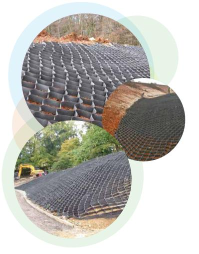
TERRAM Geocell load platforms, once filled with a free-draining granular material, act as a mattress that spreads traffic loads laterally to reduce vertical deflections. The fill is confined within the individual cells by hoop stress.
