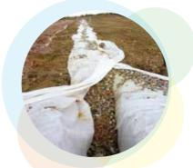
Standard Geotextiles used in a French Drain application.
