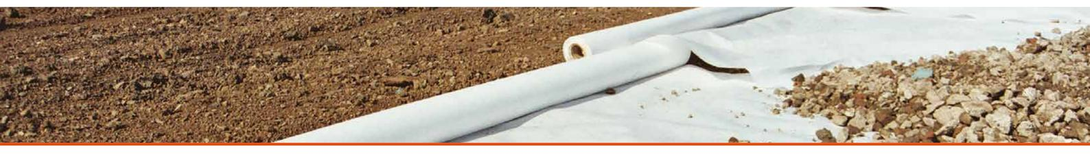
TERRAM Standard Geotextiles prevent intermixing of sub-base and subgrade layers. This intermixing causes a loss in bearing strength, as the stone layer becomes progressively contaminated, resulting in failure in the form of deformation. This can be remedied if it's an unpaved area/road by filling the ruts but even this can be uneconomic or unacceptable if stone has to be imported over long distances at a later date.
