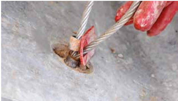
1. Position trough on a level flat area. Fix in lifting loops to each of the four lifting points. Check loops are secure.
