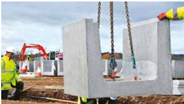
3. Ensure lifting chains are symmetrical then begin lift.
