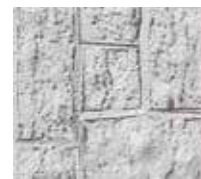
ROCK FACE SEMI-DRY
