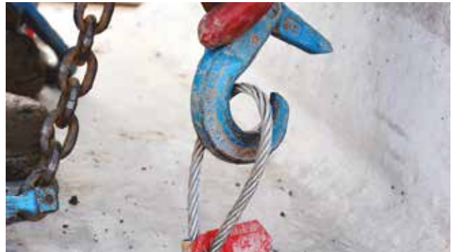
2. Attach lifting chains to all four lifting loops.
