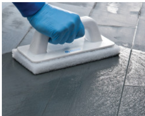
Cleaning the joints with a ScotchBrite® pad (when the product is semi-hardened)
