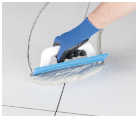
Spreading Ultracolor Plus on porcelain floor tiles with a rubber float
