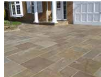
>> ProJoint™ V75-WT (neutral/buff) used on an Indian sandstone driveway
