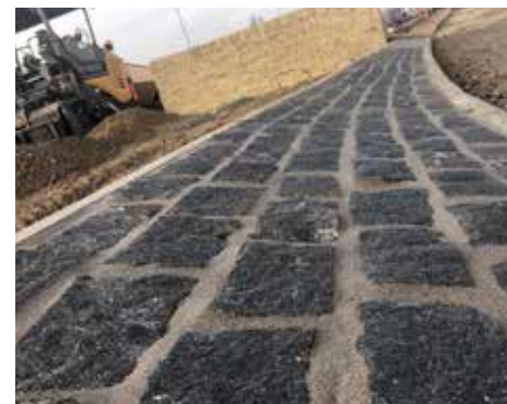
▲ ProJoint™ V400-WT (mid grey) used at the Leeds M1 Skelton Lake motorway services (see page 46)
