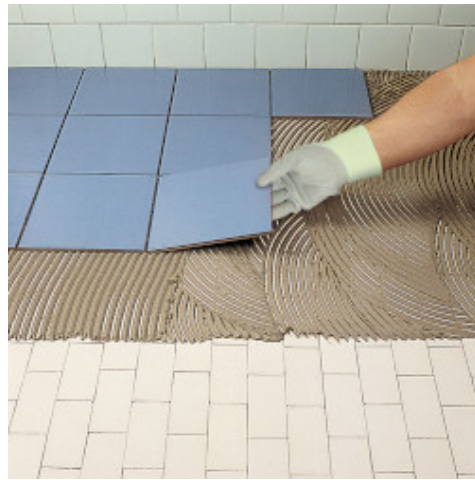
Tile on tile with Keraflex grey
