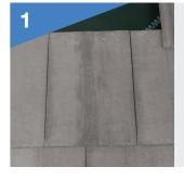
Set out the roof and lay the tiles in line with the manufacturers fixing instructions until you reach the area where the vent tile is to be fitted.
