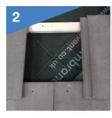
Remove the tile where it is to be replaced with an Ulti-Line Tile Vent and Mark the cut line as shown.
