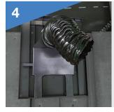
Select the Vent Tile to match to profile and colour and fit either without a flexipipe (if just being used for roof ventilation) or with a Ulti-Mate<sup>®</sup> Flexipipe ULTI3FP for connection to Soil Pipe of Mechanical Extraction.
