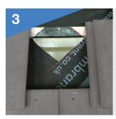
Cut the underlay as marked out and lift the cut sections with top section this is to the fixed to the batten above the opening.
