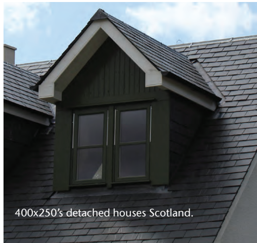
Complicated roof design requiring a versatile slate.
