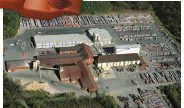
One of three large concrete roof tile factories in Germany
