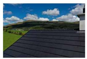
The Shetland<sup>®</sup> is unique from other similar clay roof coverings – it has been robustly designed and tested with the harsh UK and Irish climate in mind. The Shetland also has a generous batten gauging tolerance of 40mm which eliminates labour and wastage when fitting.
