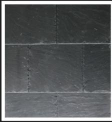
A mid-grey slate that exhibits a subtly rippled surface with a generally smooth appearance across the face overall, providing uniform thickness with a mild riven look, may contain benign surface pyrites
