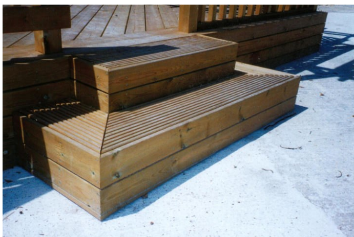
Steps can be Created by Extending Different Levels of Subframe
