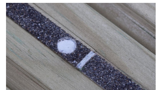
Secure the Grip Strip with a Screw
