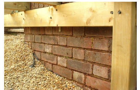
....Ledger Board Fixed to Existing Wall....
