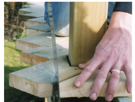
Cutting Deck Boards to the Desired Length
