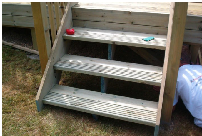
Stair Built Using Multi-Purpose String Deck Tread
