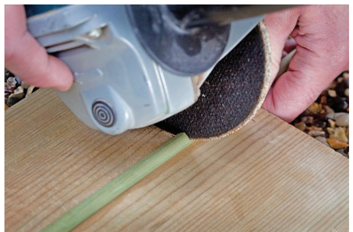
Cutting Decking Anti Slip Strips to Size
