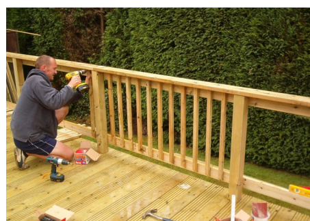
....Fixing the Balustrades....
