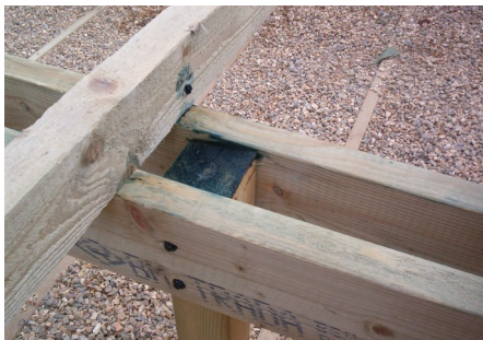
....Joist Fixed Over The Beams....
