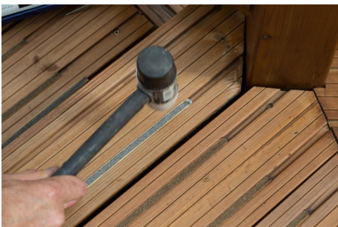
Securing the Anti-Slip Strip
