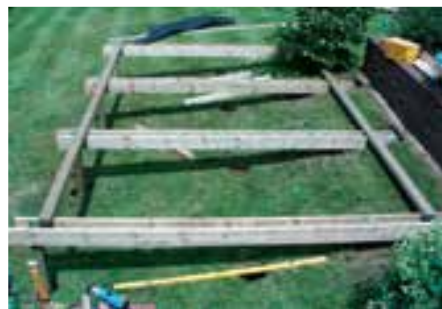
....Building the Support Beams....
