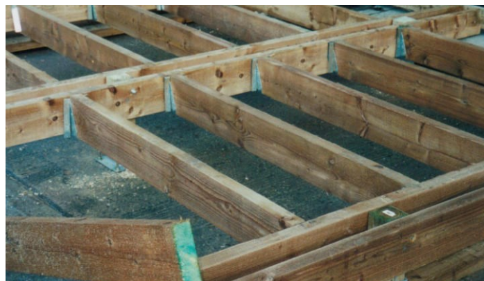
Fixing Joists to Beams
