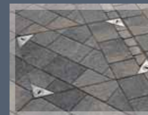
Blocks mortared into position around a cover
