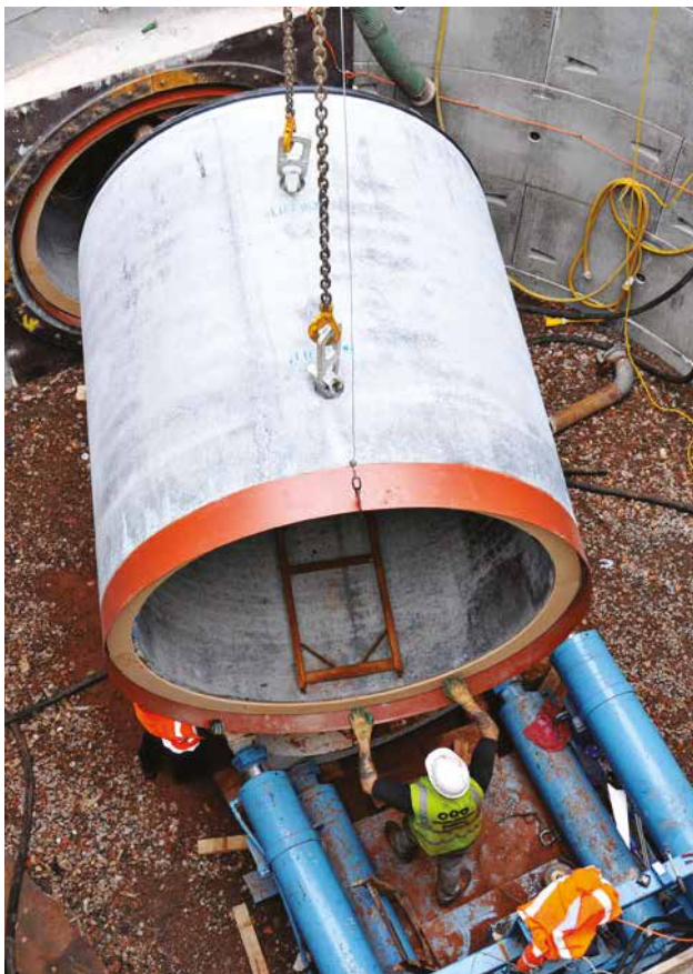
Typical position of jacks relative to pipe wall
