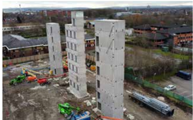
SINGLE LIFT SHAFT DOUBLE LIFT SHAFT
