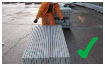
When both main bands are removed from gravel board packs the pack should remain standing when the part band is left, however will support the front board initially when opening fully (as shown above).
