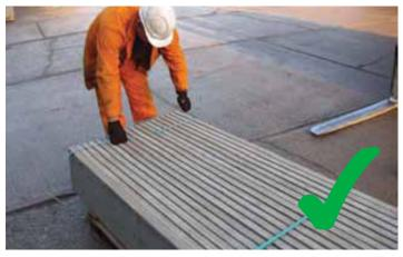
Care and attention must be paid when opening gravel boards, always leave the band holding just part of the pack, this will prevent the whole pack collapsing when the pack is opened (as shown above).
