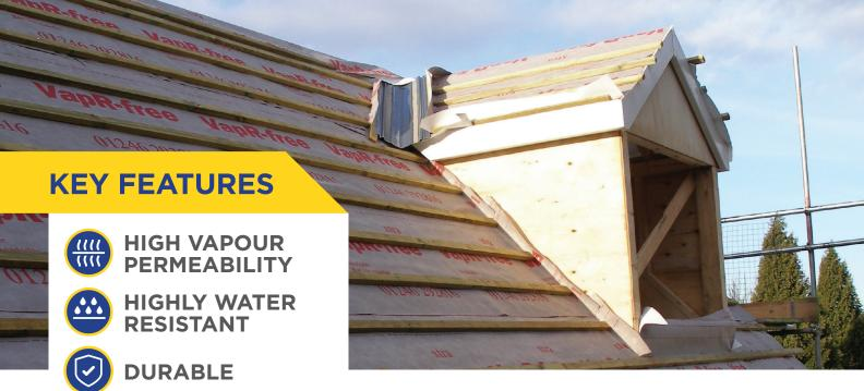
**VapR-free Xtra** is a multi layer laminate film composite made of polyolefin materials, resulting in a pitched roof underlay that has high vapour permeability, but is also highly water resistant.
