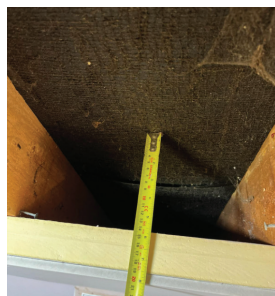
Example: cross flow ventilation to an untreated Room in Roof.
