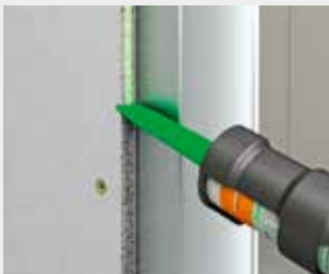
Figure 4: Guide the Greenline Jointstik along the edge of the board. The special nozzle releases the exact amount of adhesive for 10 and 12.5 mm boards. The nozzle must be cut for 15 and 18 mm boards.
