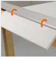
Figure 2: Breaking the section / cuttings
