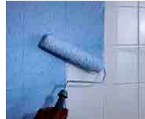
Febond Blue Grit is a high performance, plasterers grip coat bonding agent specifically designed to provide an improved key to smooth surfaces. Containing a fine aggregate, it provides a mechanical key to backgrounds such as plaster, concrete, painted surfaces, textured surfaces and ceramic tiles. One coat application, coloured blue to indicate coverage.
