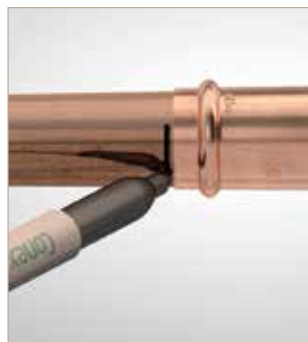
6. Assemble and mark the insertion depth
