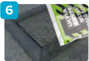
Surface finish with UltraCrete Instant Road Repair® cold lay asphalt concrete if located on a footpath, or category 3 & 4 road.
