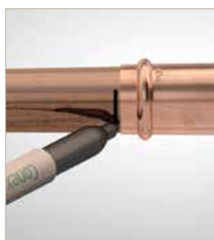
6. Assemble and mark the insertion depth
