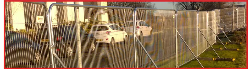
Altrad Generation are one of the biggest providers of Temporary Fencing and can offer the most effective and economic solutions for Temporary Fencing and Barriers for site boundaries. Easily locking together, both fencing and barriers can be quickly erected on site to provide a safe and secure temporary boundary. A full range of additional components can also be supplied; such as pedestrian and vehicle gates extensions and stabilisers.
