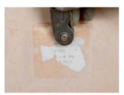
Allow plaster to adequately dry, the bead can be painted over either prior to cut-out or after.
