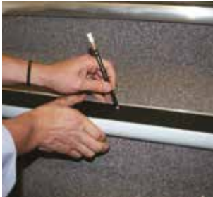
2 Position the profile, check the fit and mark the drill holes.
