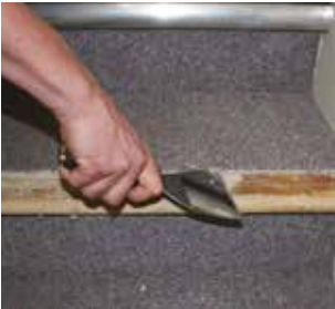
1 Prepare surface, it must be clean, smooth and free of debris.
