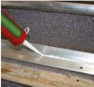
4 Apply adhesive as per manufacturer's instructions.
