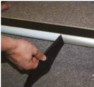
8 Remove protective film when applicable.
