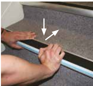
3 Position, press and slide to ensure full bond.
