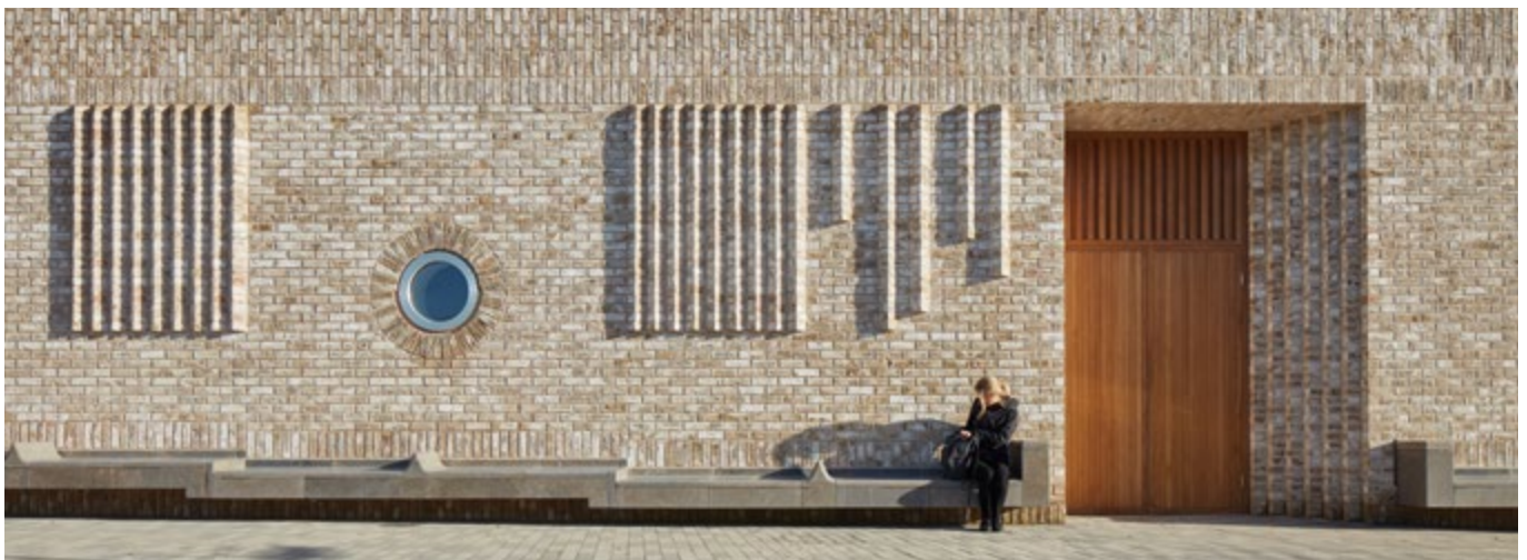
Storey's Field Community Centre and Nursery, Eddington, Cambridge CON MOSSO
