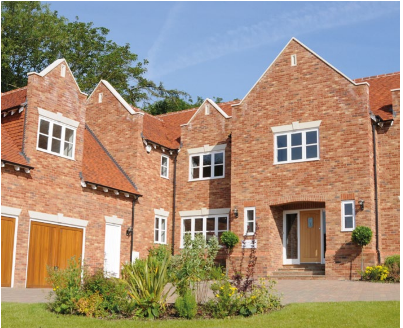
Private residence OLDE FARDALE MULTI
